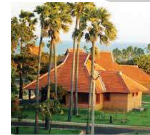
Cottage & Allied Facilities at Vivekananda Kendra, Kanyakumari
