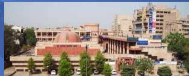
August Kranti Bhawan at Bhikaji Cama Place, New Delhi
