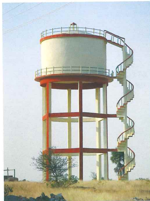
Water Tank, Nalgonda, Andhra Pradesh
