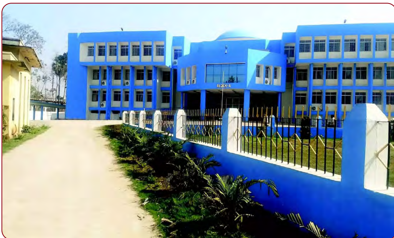
Collectorate Building Daltonganj, Jharkhand
