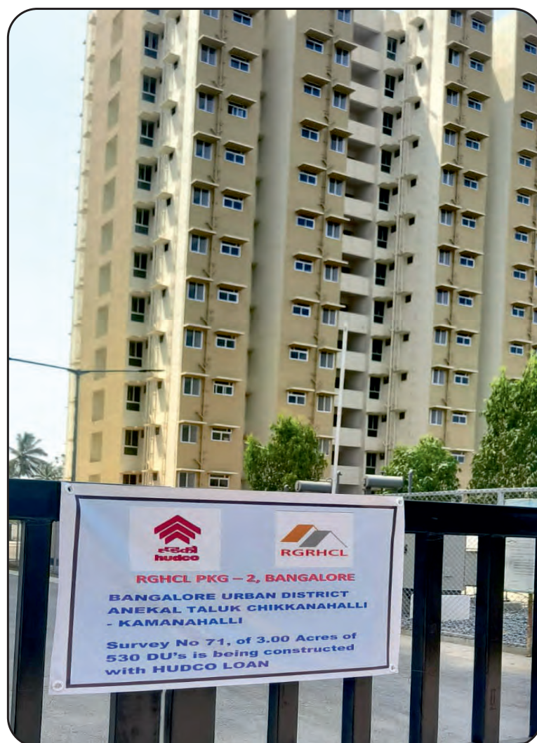
EWS Multistorey Housing Programme Bengaluru, Karnataka
