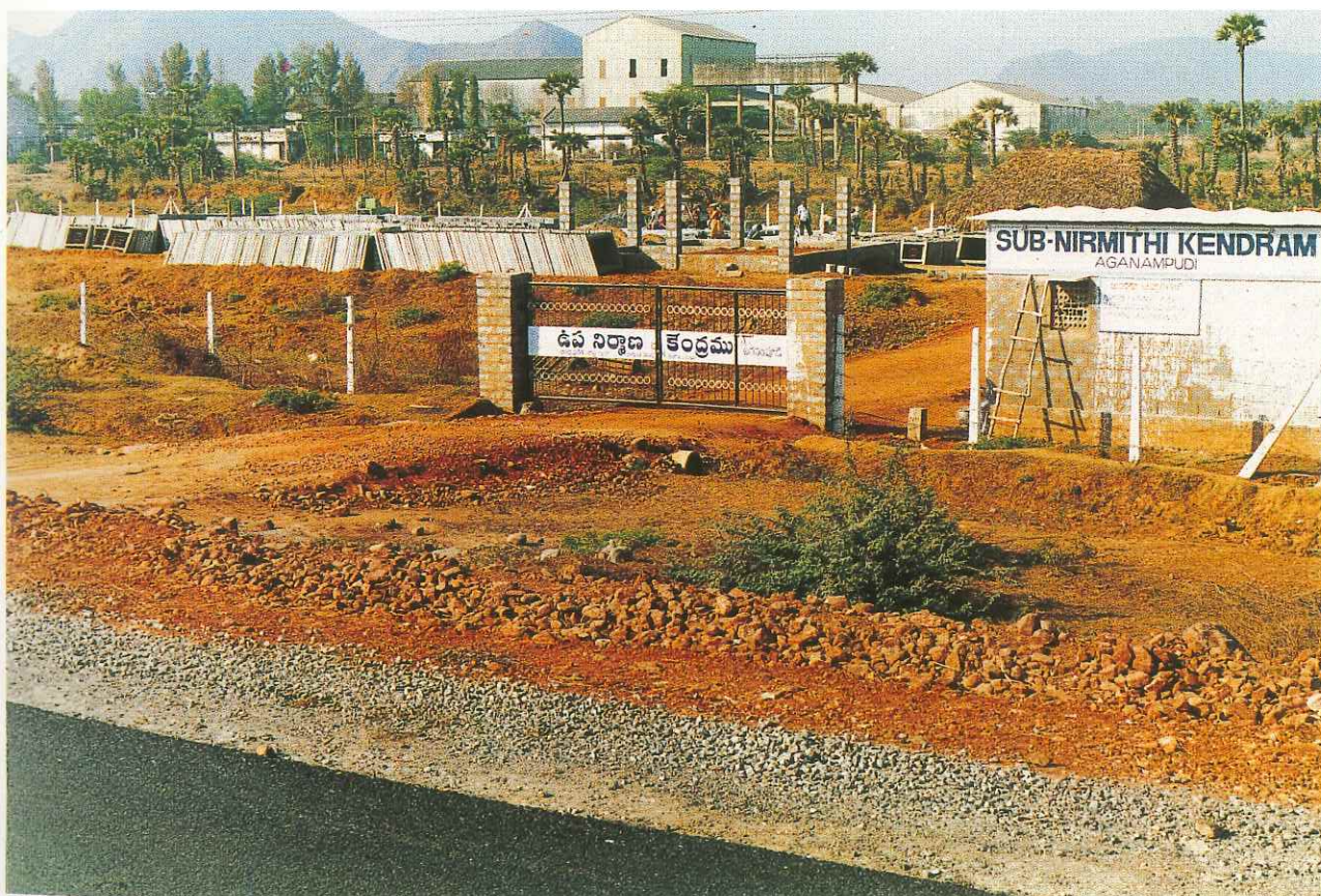
Nirmithi Kendra, Aganampudi, Andhra Pradesh
