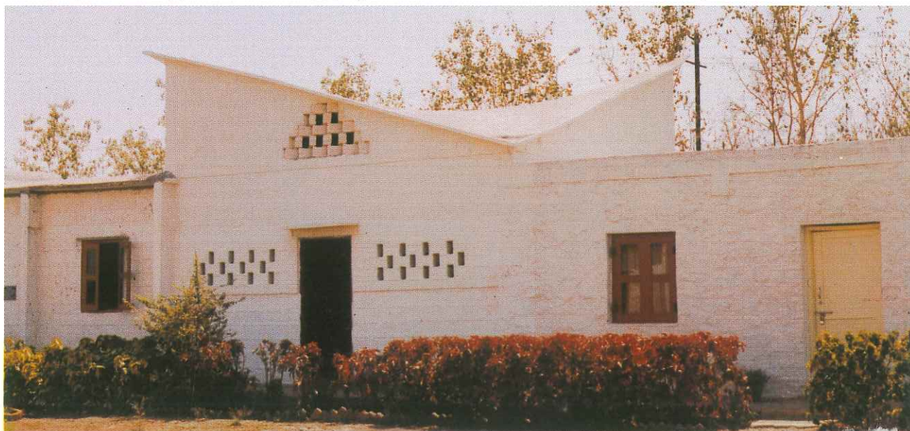
Building Centre, NICMAR, Balwadi at Pune, Maharashtra
