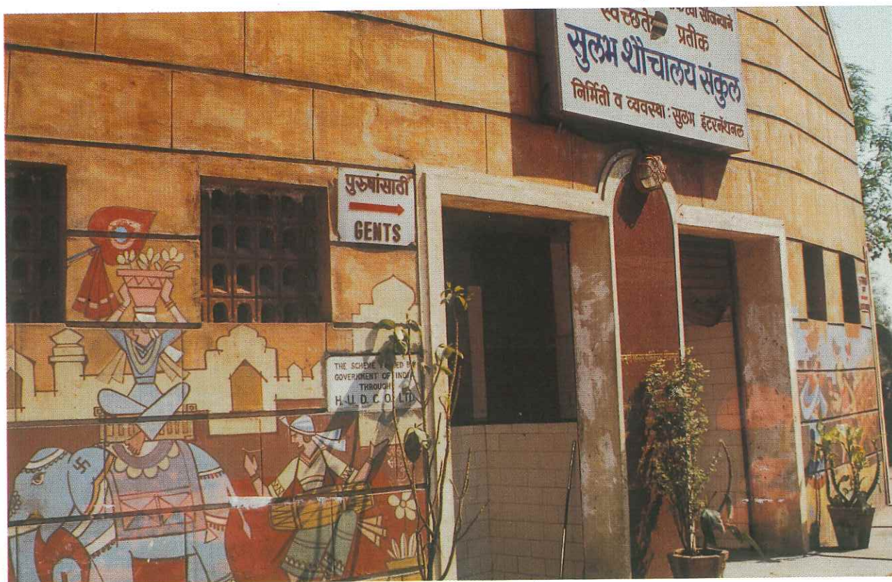
Pay & Use Toilet by Bombay Municipal Corporation, Mumbai, Maharashtra
