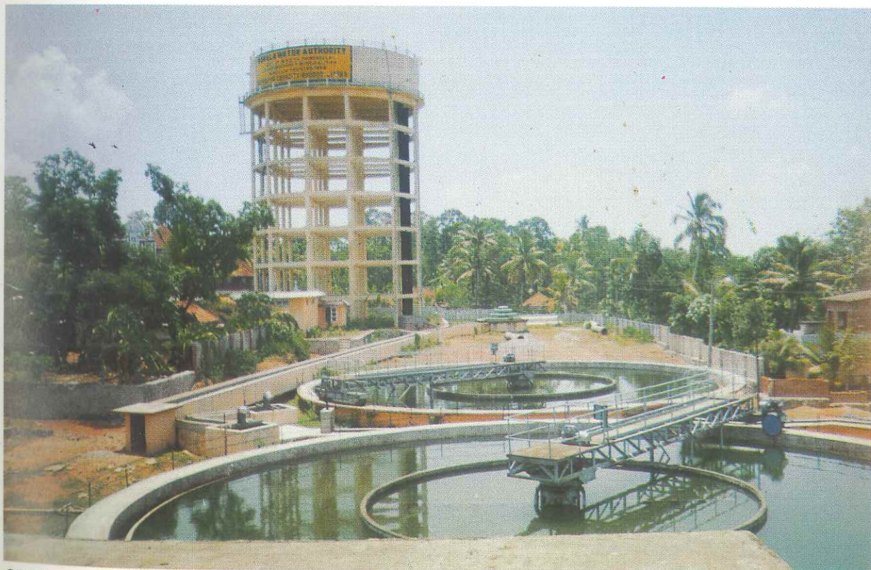
Clari Flocculator and Over Head Tank at Thiruvalla, Kerala
