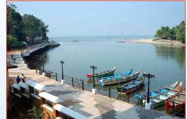
Construction of Walkway at Mahe
