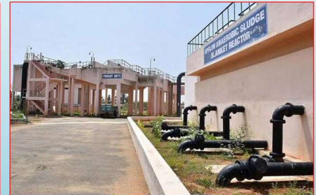
UG drainage system at Puducherry town.
