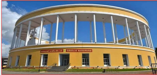
Construction of Kamarajar Manimandapam, Puducherry
