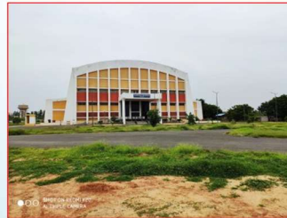
Construction of Indoor Stadium, Karaikal
