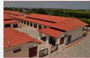
Renovation of Govt. Guest Houses in the UT
