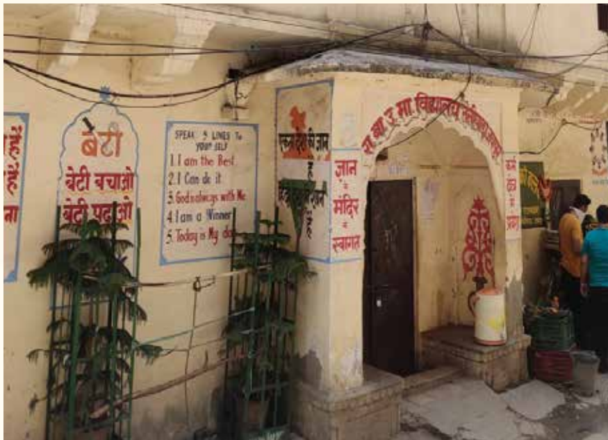
Image: Sen Sec. School Telipera- Restoring intricate carving and architectural elements to maintain authenticity
