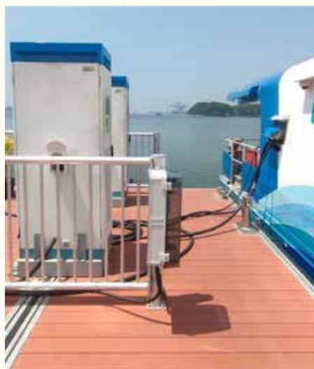
Image: Boat charging and chargers installed atop floating pontoons
