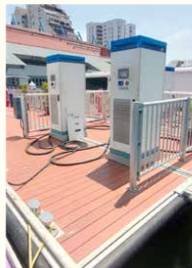
Image: Boat charging and chargers installed atop floating pontoons
