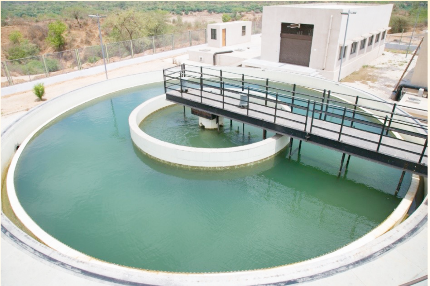
Image: A view of the a project component
