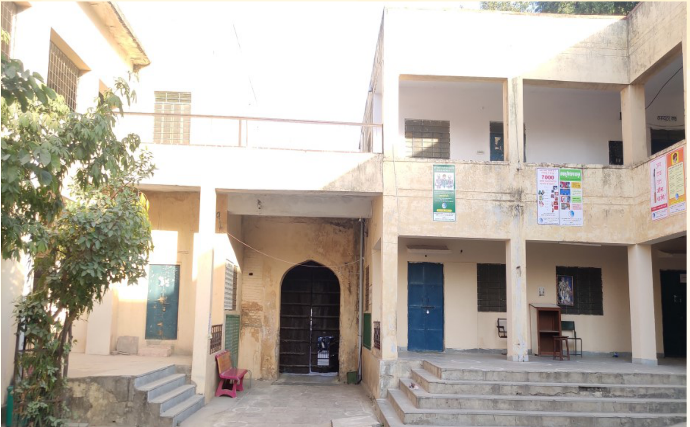
Image: Gangouri Bazar School- Restoring original architectural elements using traditional materials and techniques
