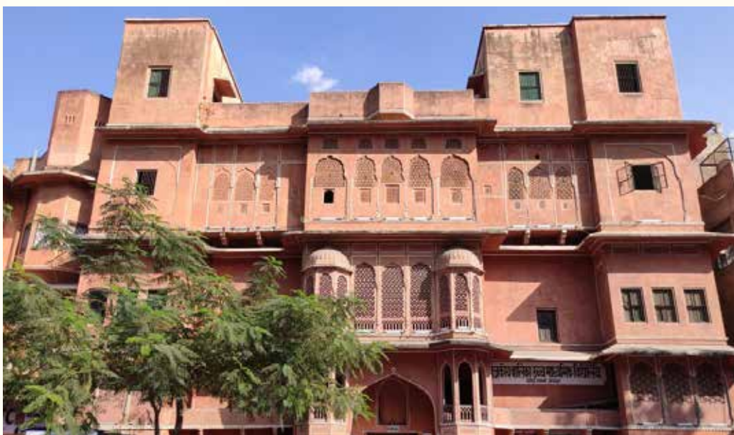
Image: Sen Sec. School Chaura Rasta- Restoring intricate carving and architectural elements to maintain authenticity
