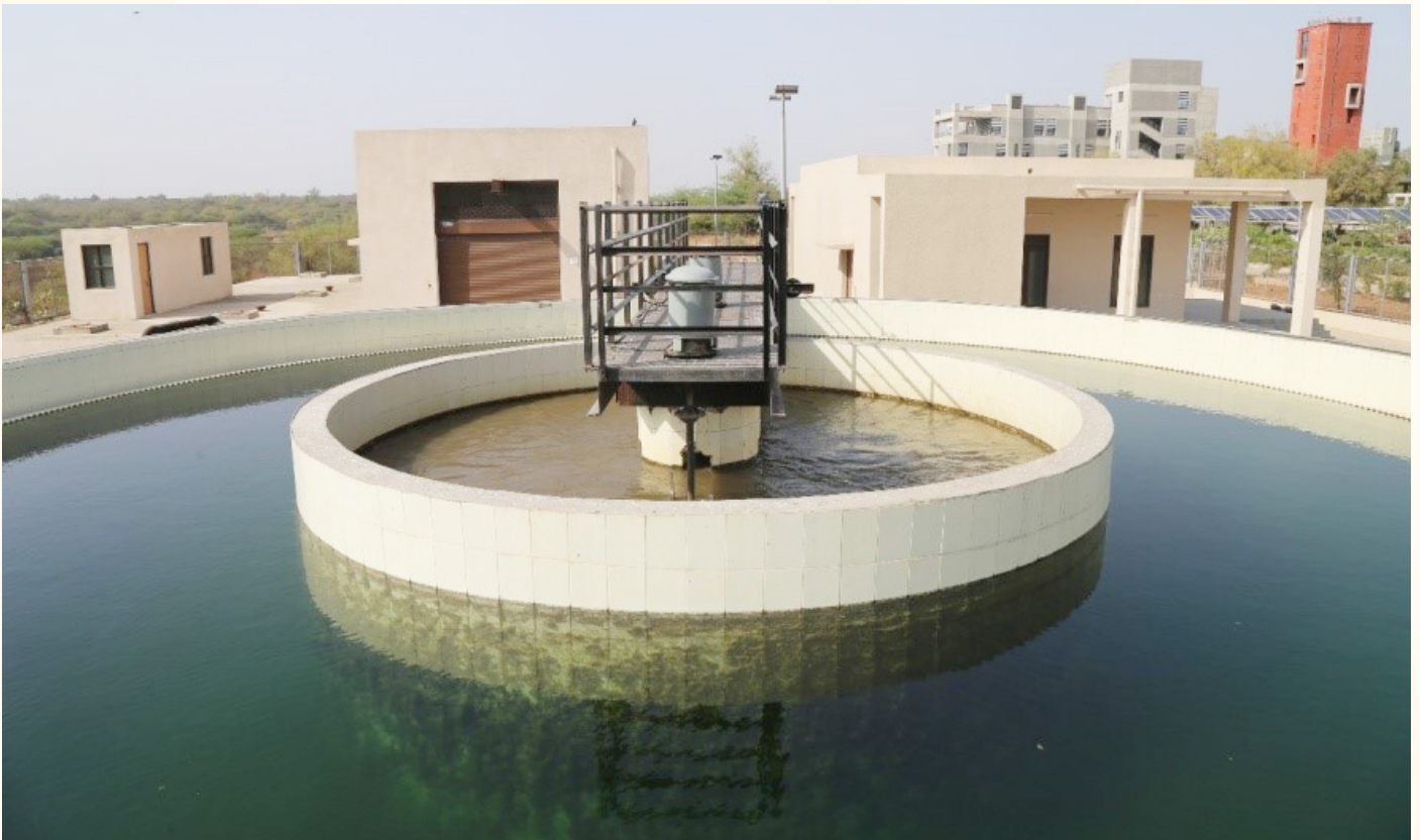
Image: A view of a project component
