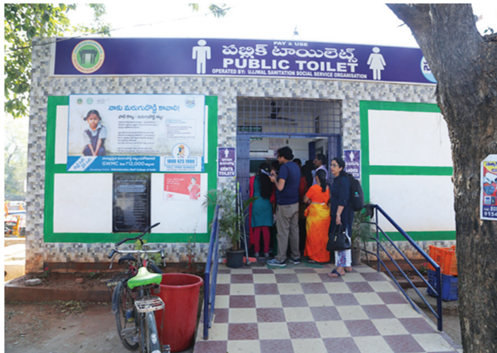
Figure 1 Public Toilet at Warangal
